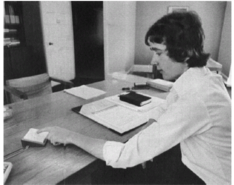
Figure 20. Low voltage switch for operating luminaires from desk
