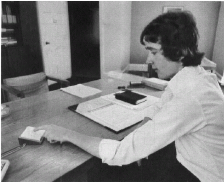
Figure 20. Low voltage switch for operating luminaires from desk
