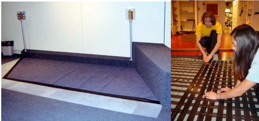
Figure 3-3. The Magic Carpet Installation at the Boston Museum of Science (left) and taping of the piezoelectric wire to the bottom of the carpet (right) before installation at the MIT Museum
