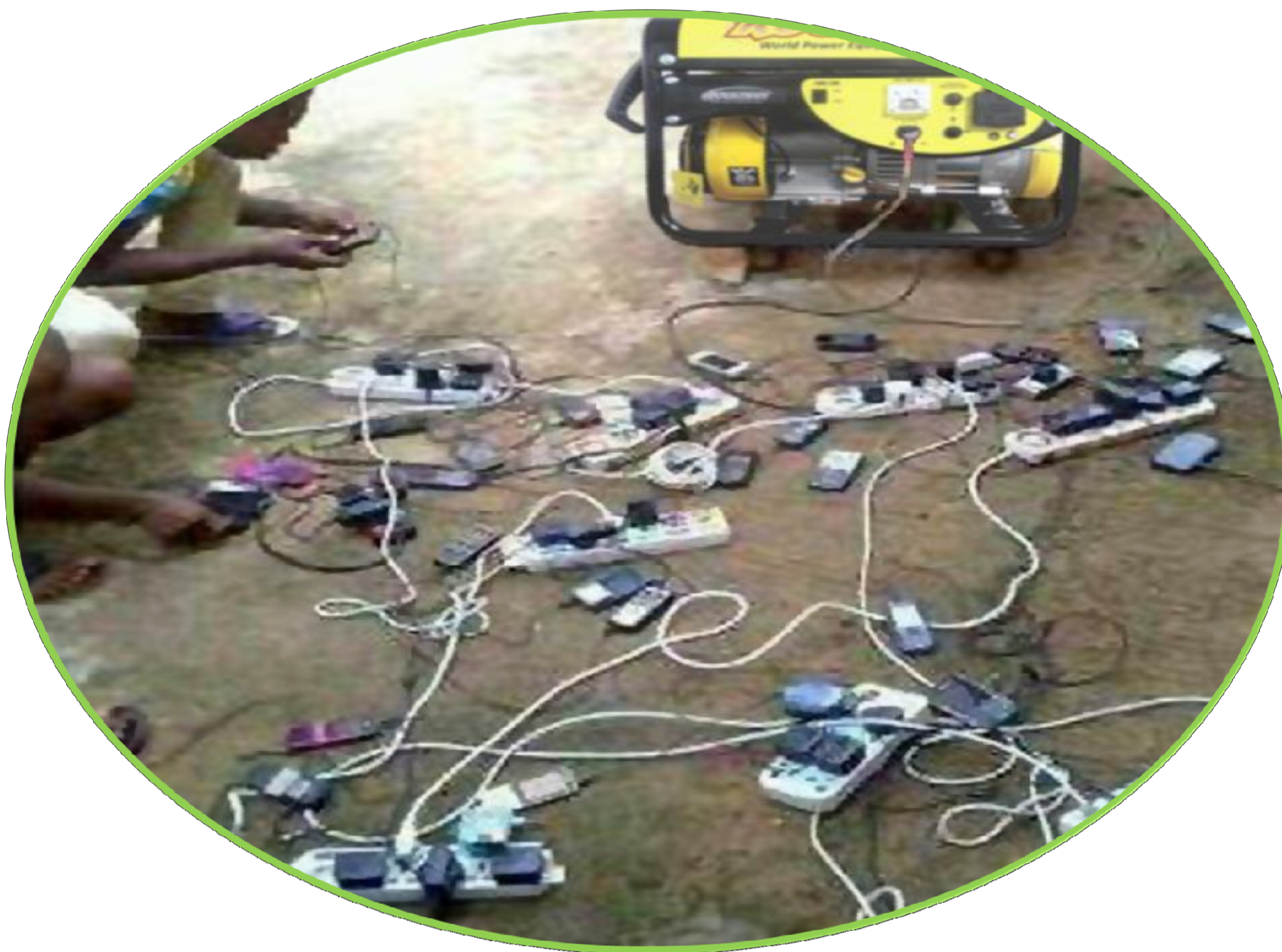
An ad hoc nano-grid used to charge cell phones.
