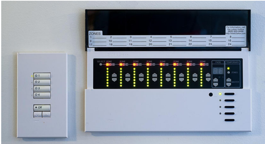
Figure 1.1: Example lighting interface to control preset “zones” of lighting found in MIT Building E14 (Image credit: Brian Mayton, MIT)
